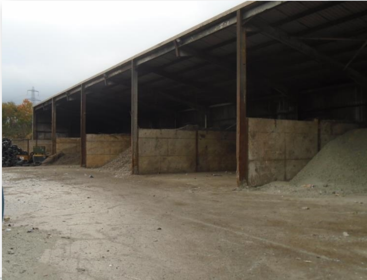
Existing building to be demolished
