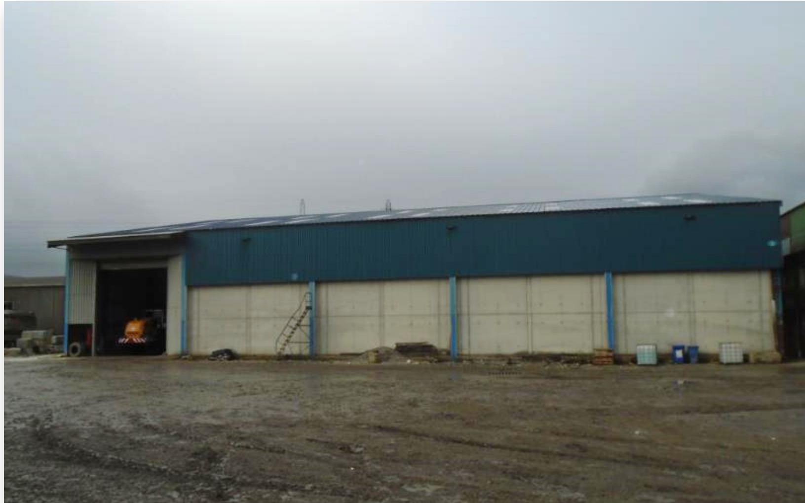
Building B in front of application site
